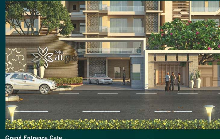
Grand Entrance Gate
